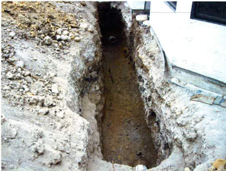
Figure 19: Trenching to repair pipes improperly installed from original installation
