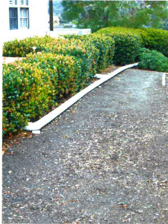
Figure 49: Temporary drain lines to be placed underground 2nd of 3 locations
