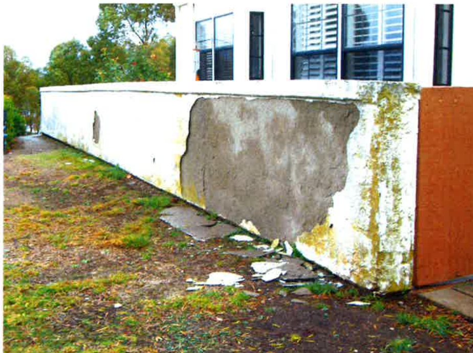
Figure 21: Deteriorated Stucco
