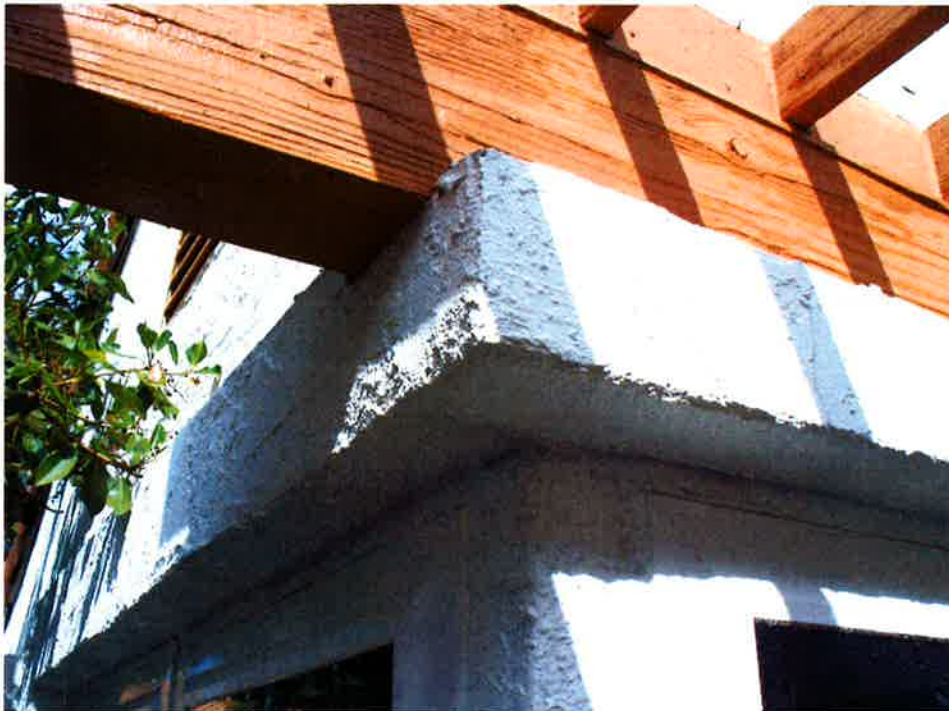
Figure 57 Pop-out and trellis beam above front elevation windows
