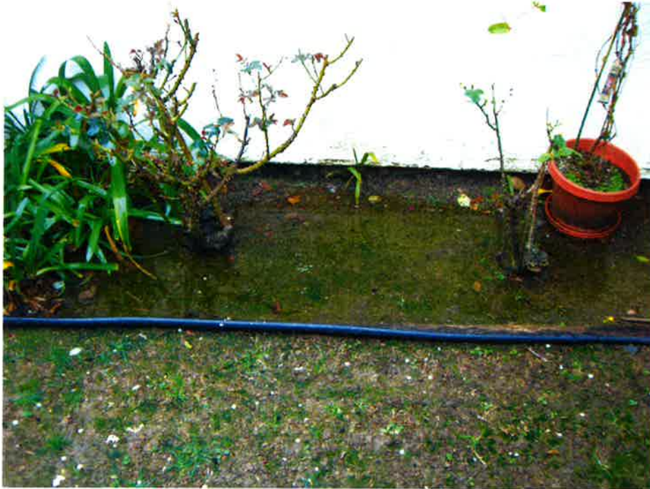
Figure 44: Ponding by side of garden wall
