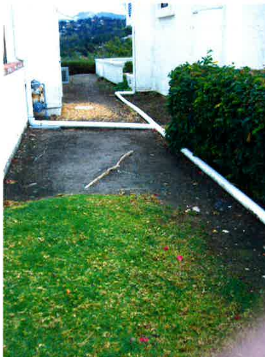
Figure 48: Temporary drain lines to be placed underground 1st of 3 locations
