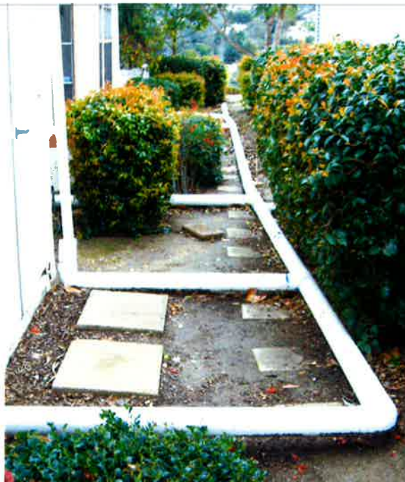
Figure 50: Temporary drain lines to be placed underground 3rd of 3 locations
