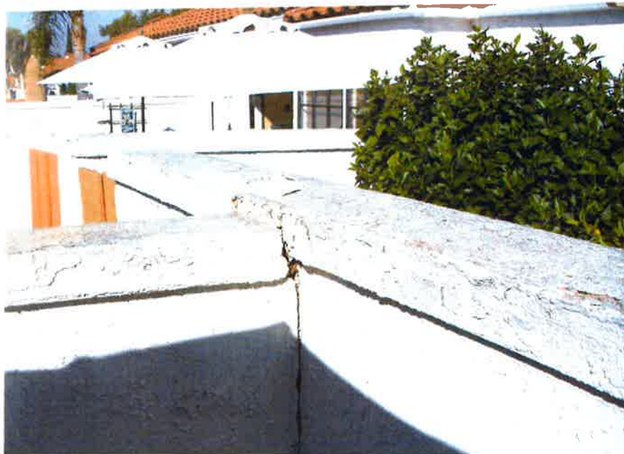
Figure 25: Rotted post resulting in wall setting
