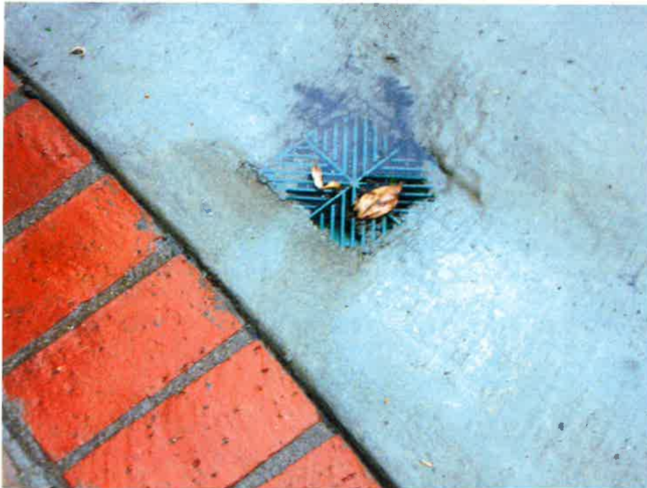
Figure 45: Clogged drain
